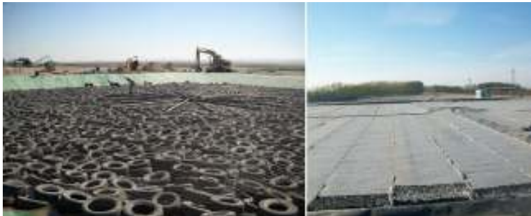
31,000 tires installed (left) and digester cover in place (right)
